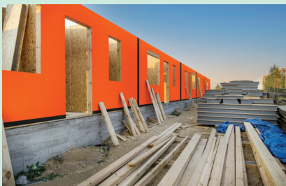
Above: Arclin promoted its Arctek Dryshell factory applied protective, vapour control overlay for timber construction panel products
